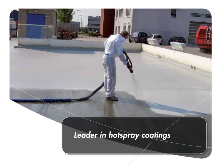
Prokol specialises in the development and production of polyurea, polyurethane, and hybrid hotspray coatings. These Rocathaan hotspray coatings are applied hot using special spray equipment.
